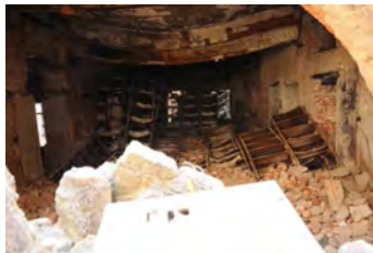
Fig.4 Steel beams elongated and Deflected after fire
