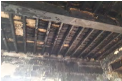
Fig.1 Wooden beams still the Madras terrace in position
