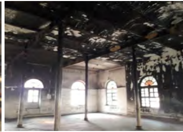
Fig.2 Wooden beams still the Jack Arch in Position
