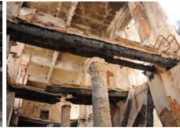
Fig.3 Wooden beams after fire
