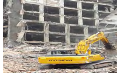
Fig.6 Inner view of Fire affected Chennai Silks
