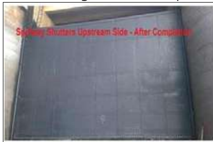
Fig. 4 : U/s of the newly replaced Gate
