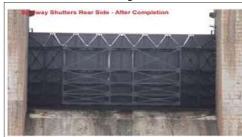
Fig. 5 : D/s of the newly replaced Gate
