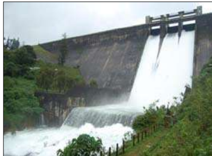
Fig. 2 : Downstream view of Sholayar Dam
