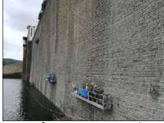
Fig. 5: Execution of Upstream face treatment using electric suspended platform
