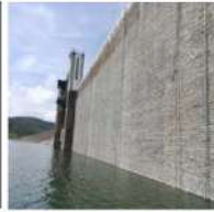
Fig. 8 : After execution of u/s face treatment
