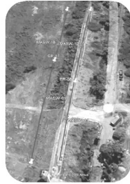
Figure 15. Right flank Earthen Embankment
