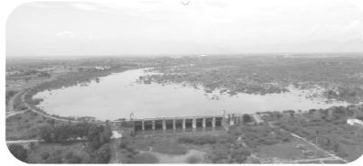
Figure 1. Aerial view of Anaikuttam Dam with earthen bund and spillway
