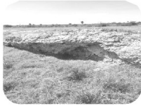
Figure 8. Kankar / calcrete strata on upstream side of the dam
